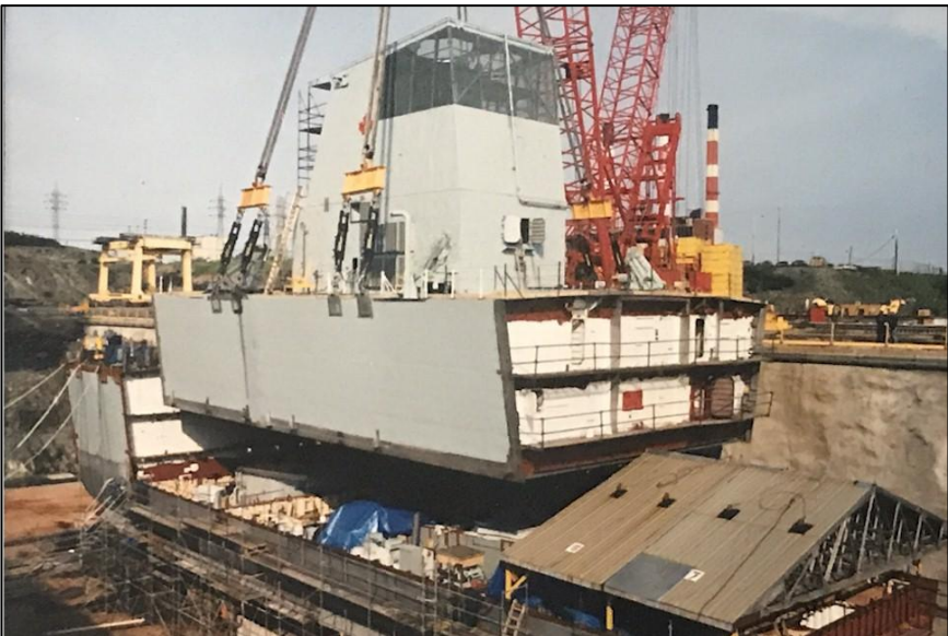
HMCS Vancouver Under Construction
